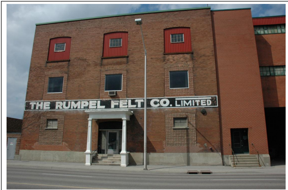
60 Victoria Street North, front elevation facing Victoria Street North
