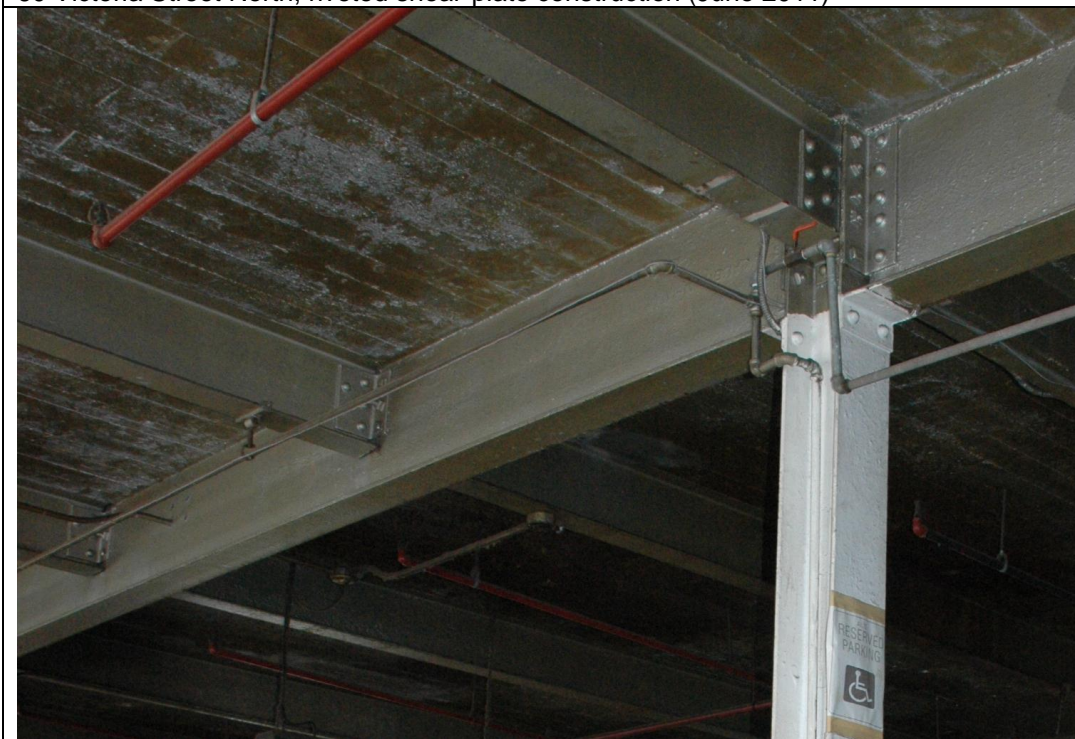
60 Victoria Street North, riveted shear-plate construction (June 2011)
