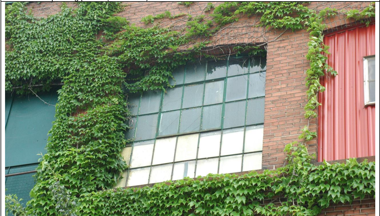
60 Victoria Street North, large-arched windows with brick voussoirs and multi-pane windows with metal mullions and pivoting panels (June 2011)
