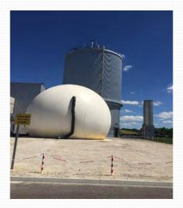
Anaerobic Digester produces valuable biogas.
