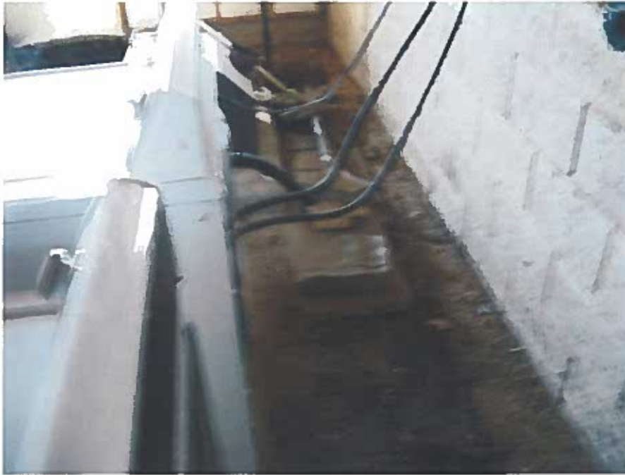
2252 Salem trench along west wall of basement & sump pump Mar 9/15
