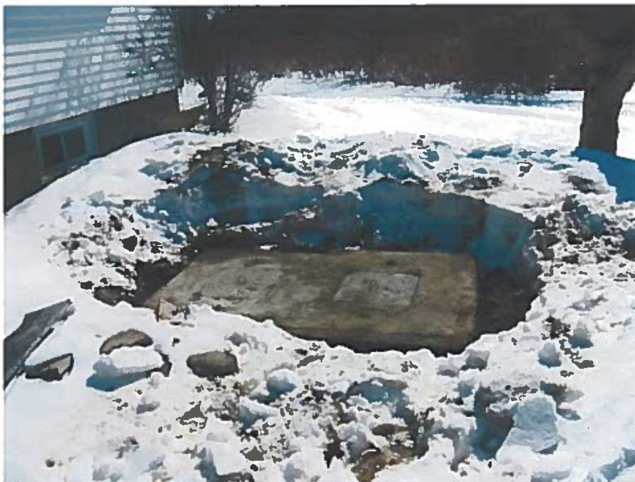
2252 Salem septic tank located near the west basement wall
