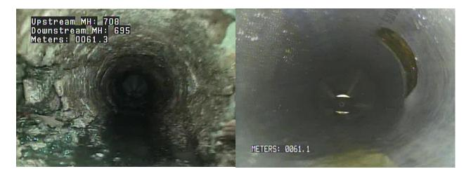
The main benefit for this innovative technology is the substantial cost savings achieved by avoiding open excavation. In a road reconstruction setting, the approximate cost for replacing sanitary sewer ranges from \$1,300 to \$2,000 per metre. Under the same generic setting, sewer lining is in the range of \$250 per metre.
