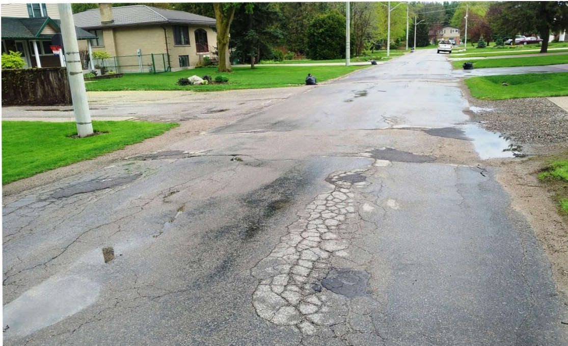
Ponding and road fatigue on Pleasant Drive, facing North toward Devon Street.
