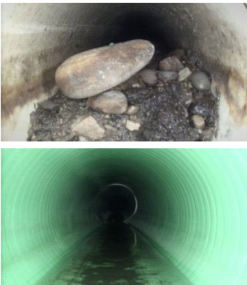
A CCTV camera is used to capture images of Cambridge's storm sewers.
