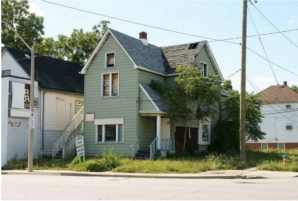
Figure 1 – Abandoned/Derelict Home in a city setting
