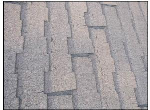
Several shingle tabs were also noted to have broken off along the west gable end of Block D at the time of our inspection. In our experience, it is not uncommon for shingles in this deteriorated condition, which become brittle, to be torn off by wind exposure that would not result in damage to sound shingles. We recommend the roofs be monitored for damage such as this to limit potential for leakage which may result.
