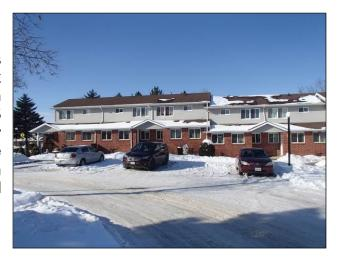
This complex includes four blocks which are identified as A, B, C, and D as shown in the Google Satellite image included below. The asphalt shingled roofing is continuous between units within these blocks (not separated by fire walls). This report applies to each block.
